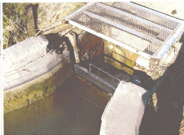
Culvert from Lake into New River
