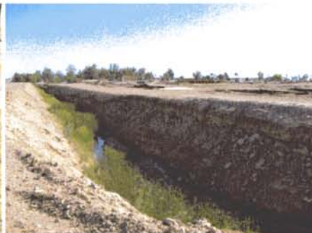
8 - Jurisdictional drainage on southwestern side of project site
