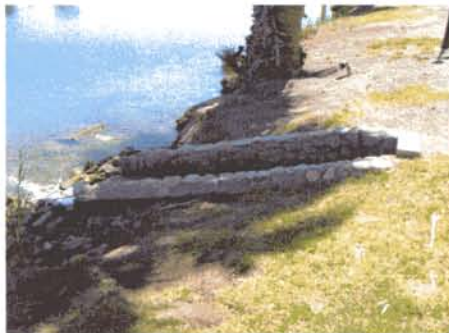
7 - Culvert into lake from pond by RV park office
